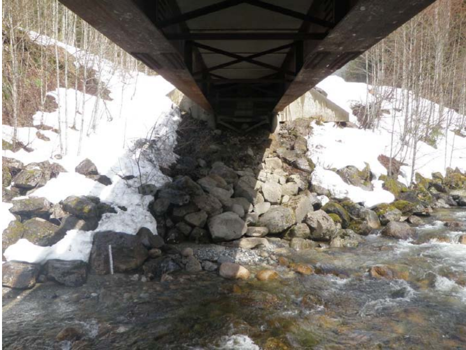
Right abutment riprap
