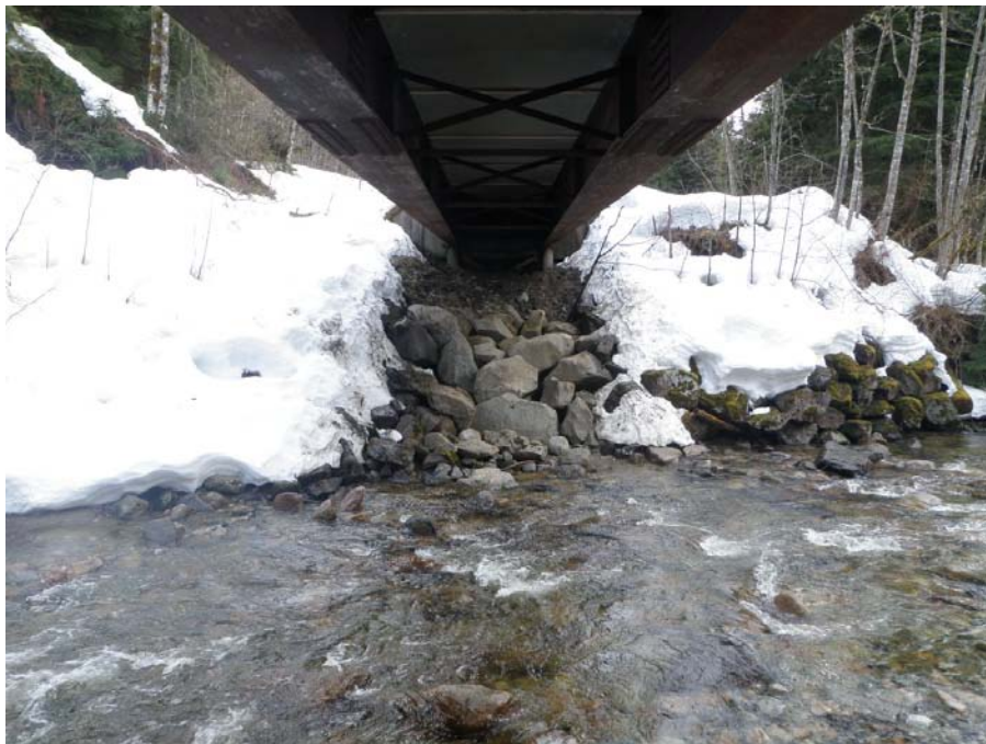
Left abutment riprap
